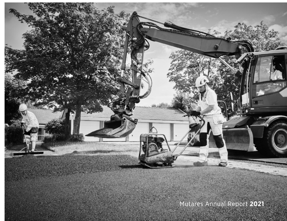
Asphalt infrastructure project in an urban area executed by a multi-skilled Terranor project team in Sweden
