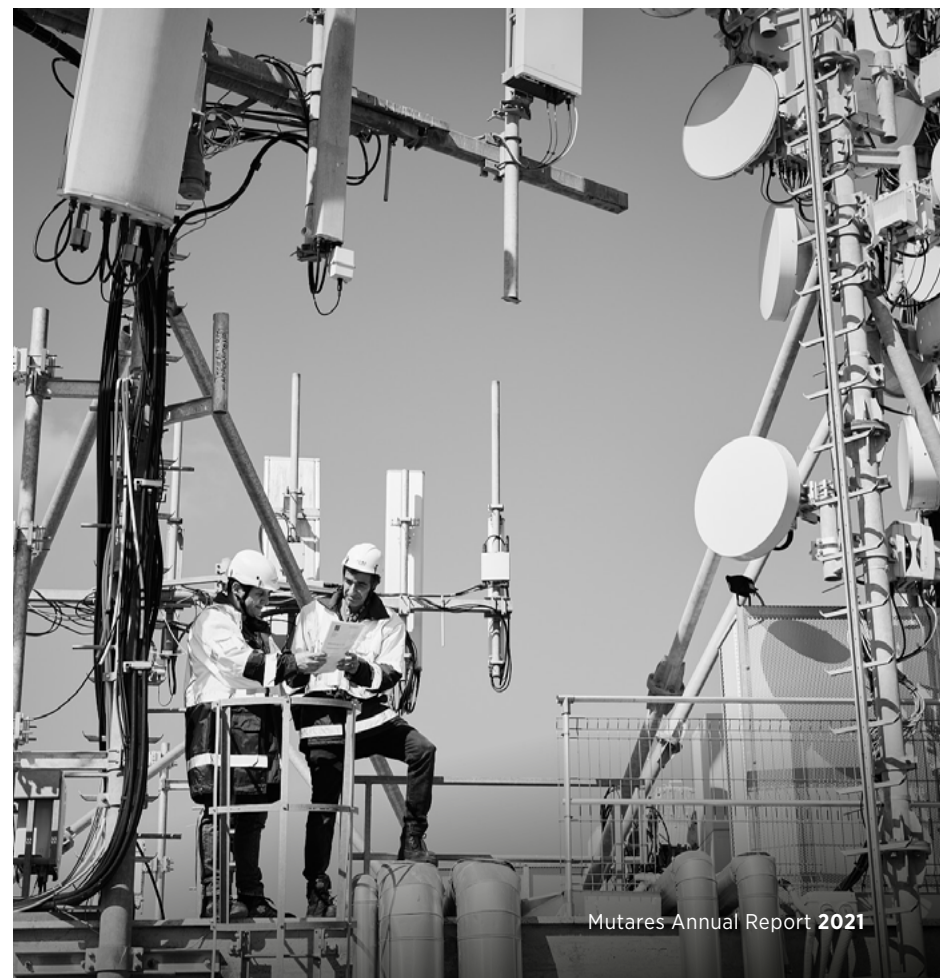
Employees during maintenance on site
